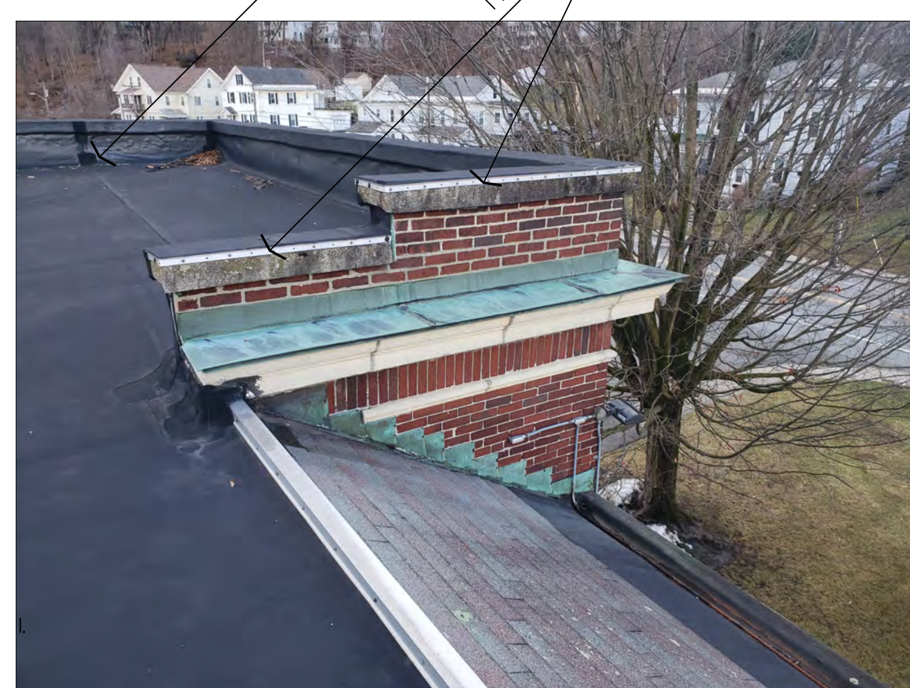
SLOPED PARAPET COPING CAP
